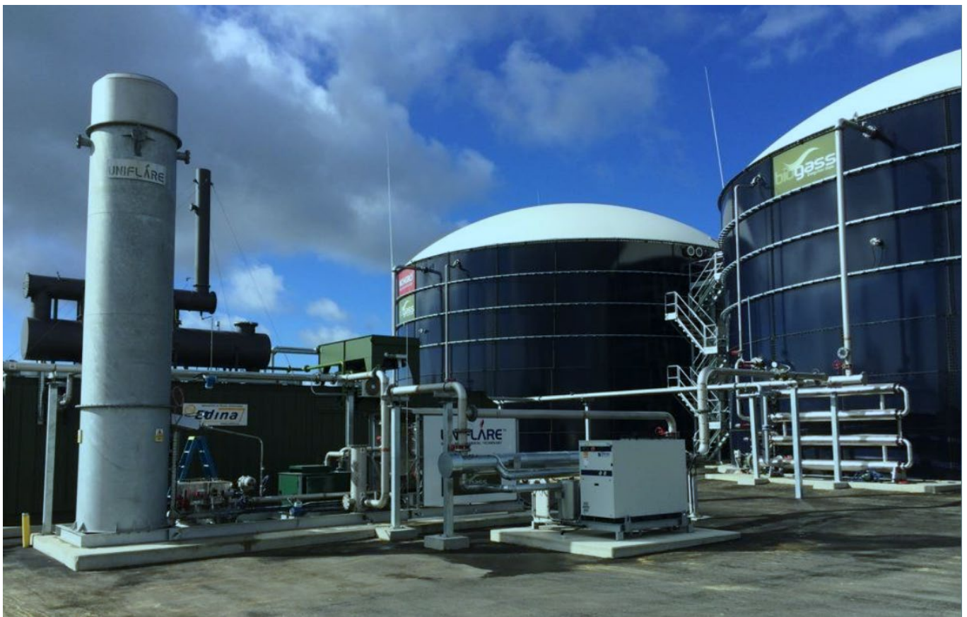
Photo 1: Richgro's anaerobic digestion facility (source: Biogass Renewables)
